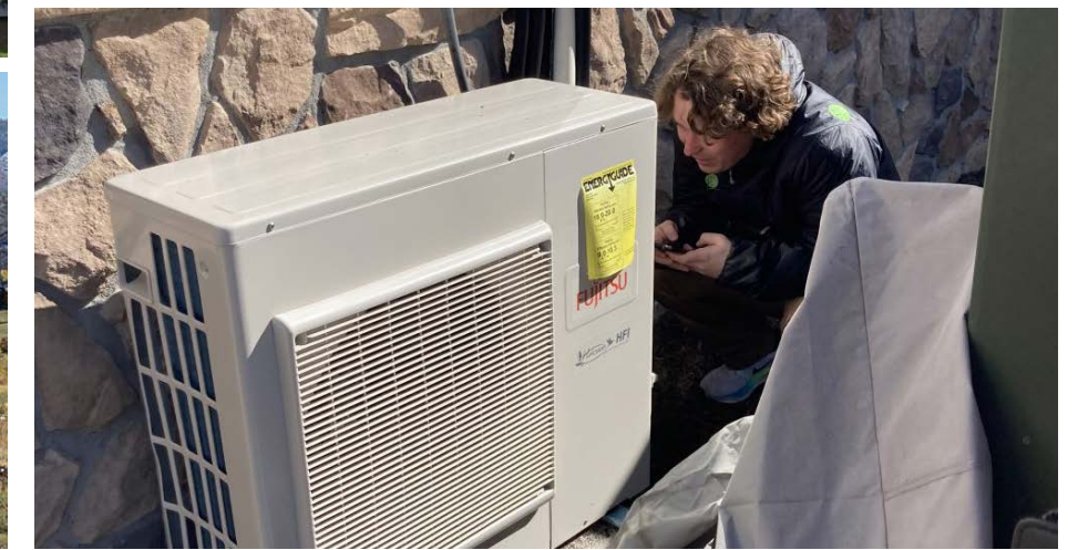
Heat pump installation in Steamboat. Source: Steamboatpilot.com
